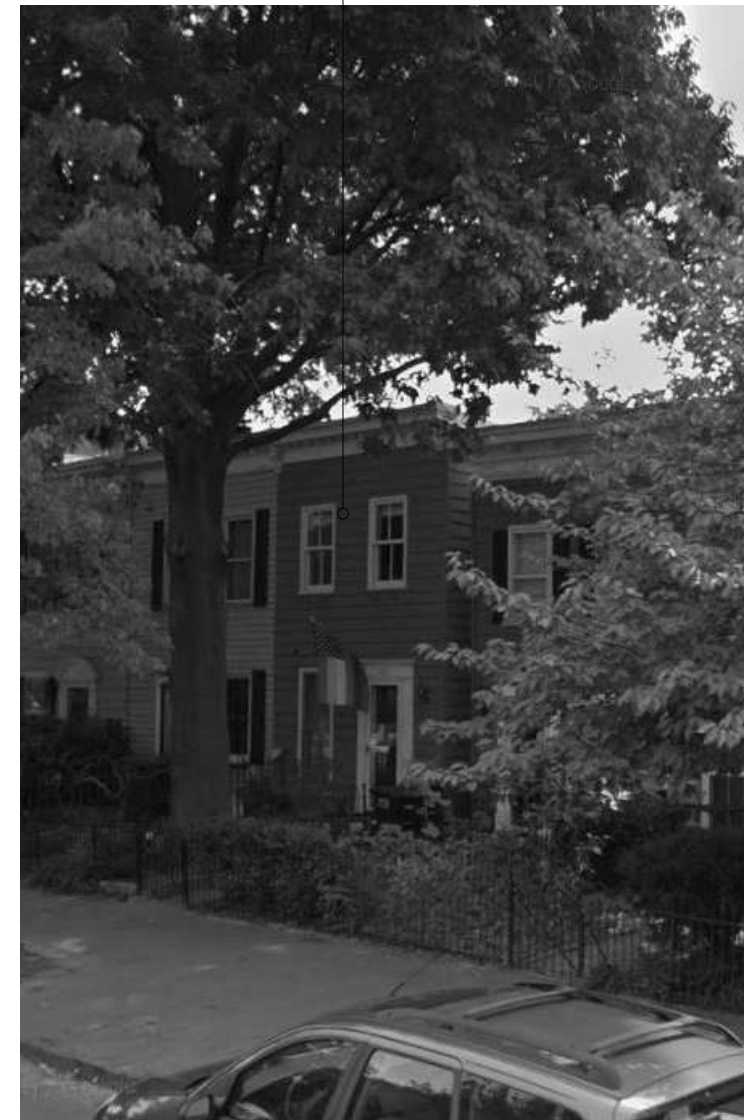
3 FRONT FACADE WEST OF PROPERTY
